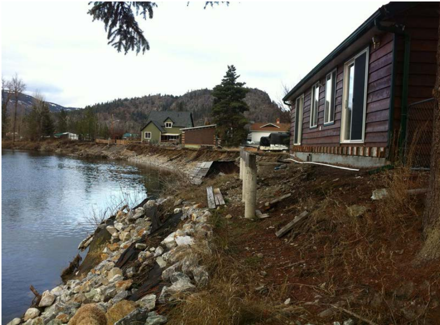
Figure 1 Structure undermined by eroded river bank, December 22, 2018 (photo from Applicant)
