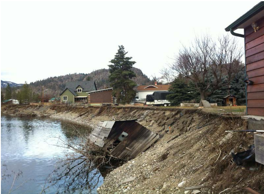
Figure 2 Structure moved by eroded river bank, December 22, 2018 (photo from applicant)
