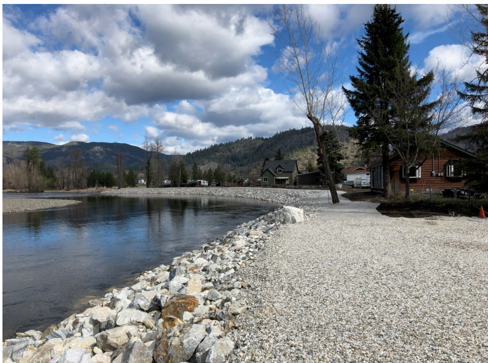
Figure 3 River Bank following rip-rap installation, looking north at 64 th Ave April 17, 2019 (photo Planning Dept.)
